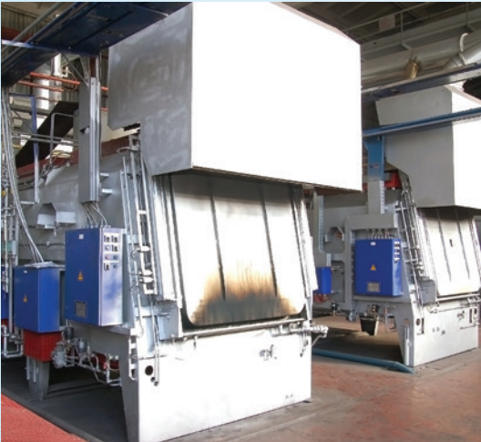
Medium scale multi-process multi-PID loop manufacturing lines
